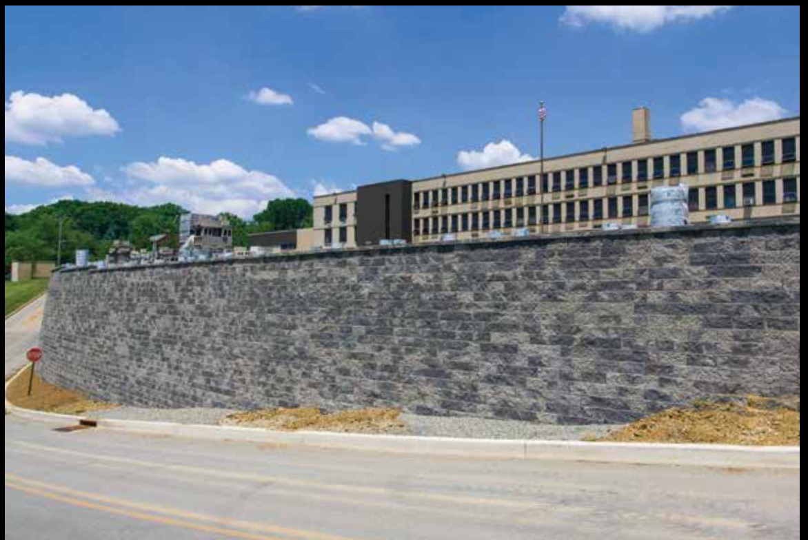
VERSA-LOK® SQ. FT. BLOCK - SLATE BLEND ALSO SHOWN: C CAP - SLATE BLEND (COMMERCIAL APPLICATION UNDER CONSTRUCTION)
