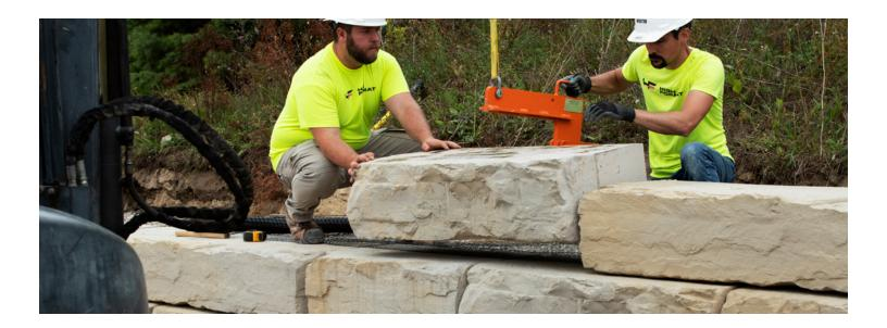
Placing the next course of blocks is similar to placing the first course. The primary difference is that you must engage the shear heels of the upper blocks with the backs of the lower blocks. Tips to accomplish this include:
