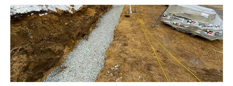
Proper base preparation is one of the most critical elements of retaining wall construction. The retaining wall is only as stable as the foundation it is placed on. If subgrade soils are deemed unstable or excessively soft, contact a qualified geotechnical engineer for remediation. The solution may entail over-excavating and replacing the soft soil with compacted granular material.
