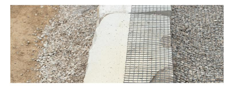
For walls that need to be taller than what is stable using an unreinforced, gravity-type structure (ie. stacked blocks), they can easily be reinforced with geogrid.
