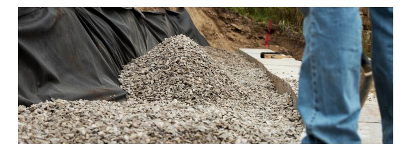
Appropriate selection and placement of backfill is necessary for the structural integrity of the wall. **Place only backfill materials which are consistent with the wall design.** For safety reasons, do not stack wall blocks more than 3 feet (0.9 meters) high before backfilling. See <u>Figure 2</u>.
