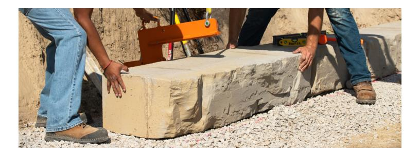
Proper placement of the bottom course of wall blocks is critical in determining the overall appearance and integrity of the finished project. Take extra time on this step and the rest of the project will go smoothly.
