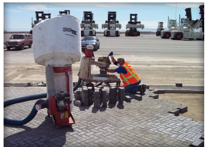
Figure 8. Saw cutting pavers.
