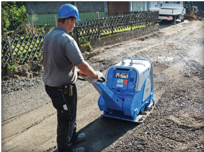
Figure 4. Base compaction with a reversible plate compactor.
