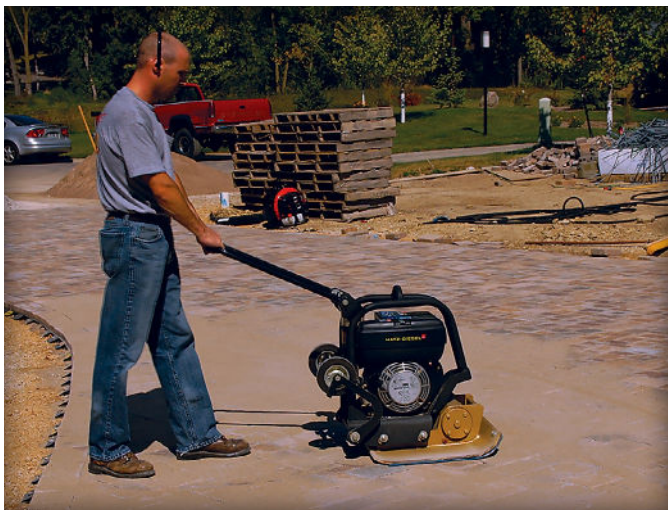
Figure 11. Vibrating sand into the joints.
