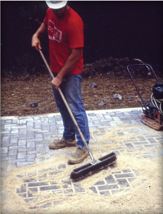
Figure 10. Spreading the joint sand.
