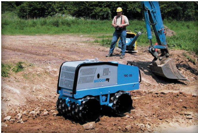
Figure 2. Compacting the soil subgrade.
