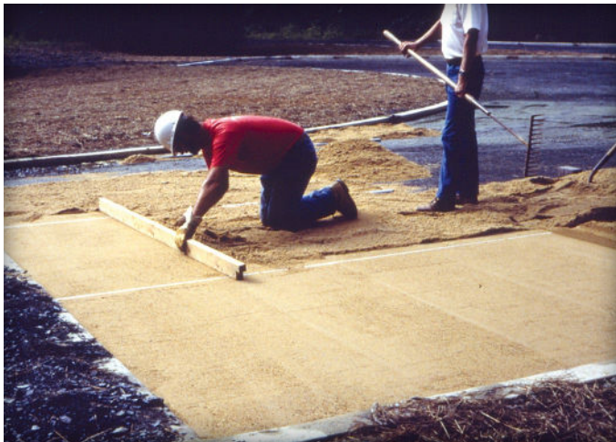
Figure 6a & 6b. Screeding the bedding sand.
