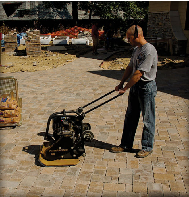
Figure 9. Compacting the pavers and bedding sand.
