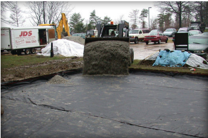
Figure 3. Application of the geotextile under aggregate base.
