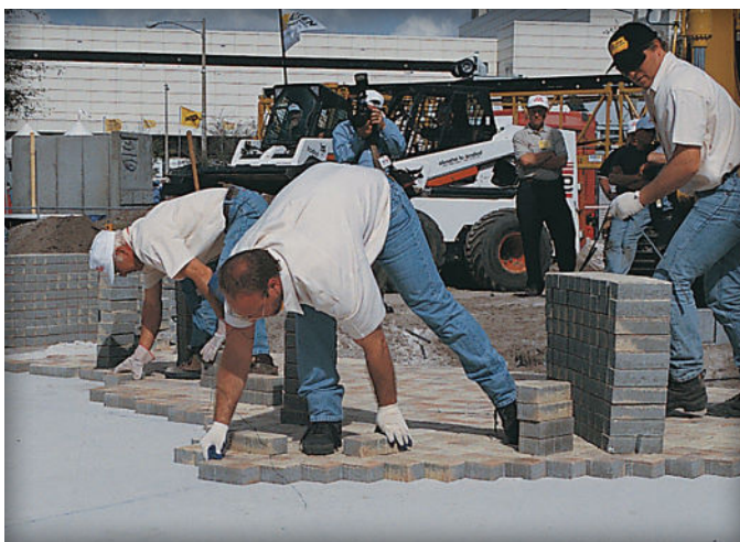
Figure 7. Placing the concrete pavers.
