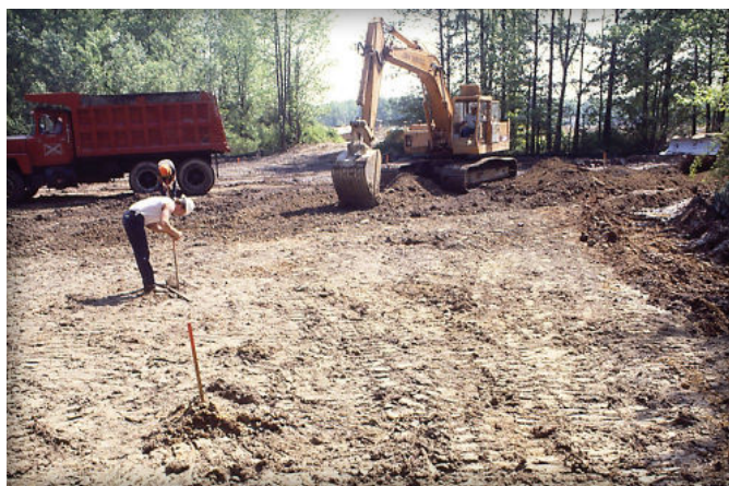
Figure 1. Excavation of the soil subgrade and placing grade stakes.
