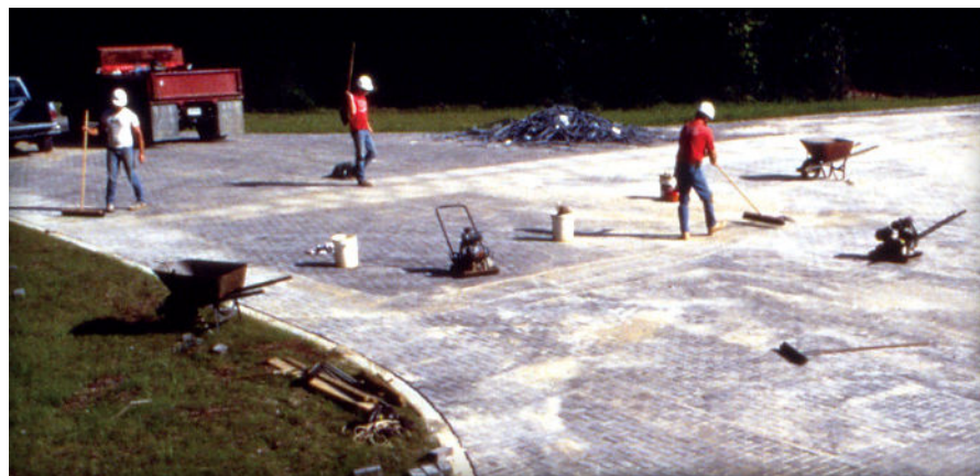
Figure 12. Removing excess sand from the finished surface will make the pavement ready for traffic.
