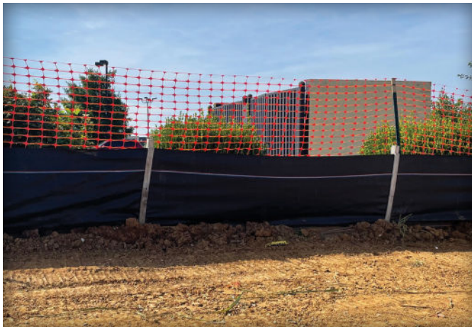
Figure 10. Typical silt fence application.
