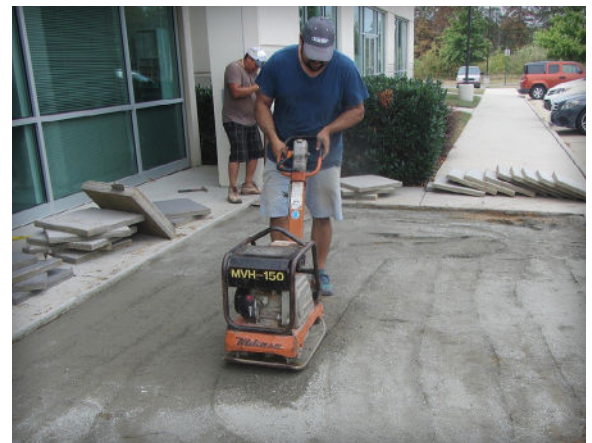
Figure 5. Precompacting the bedding sand
