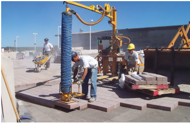
Figure 12. Self-contained vacuum lifter with boom
