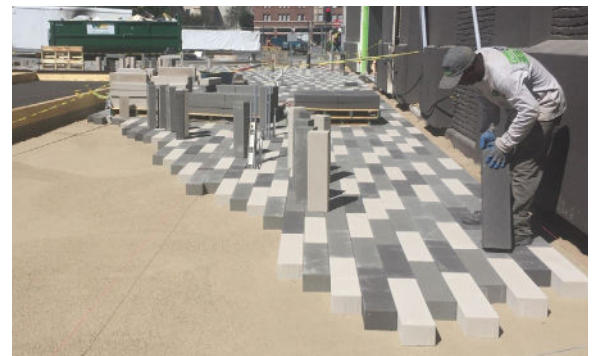
Figure 6. Installing planks on uncompacted bedding sand.
