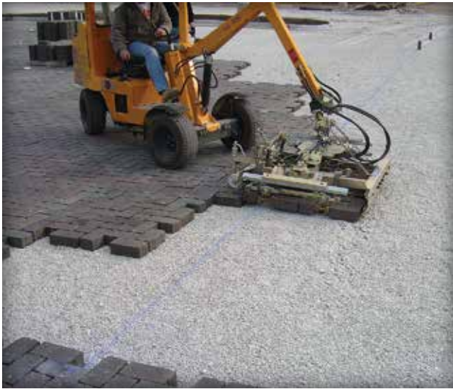
Figure 27 and 28. Mechanical equipment accelerated installation of a parking lot in Illinois and a street in Oregon.
