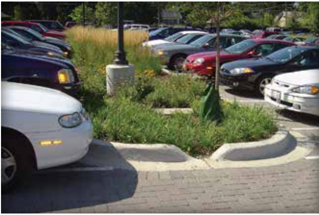
Figure 5. Elmhurst College, Elmhurst, Illinois parking lots uses full infiltration through the soil subgrade with overflows directed through curb inlets into bioretention areas and overflow drains to manage extreme rain events.
