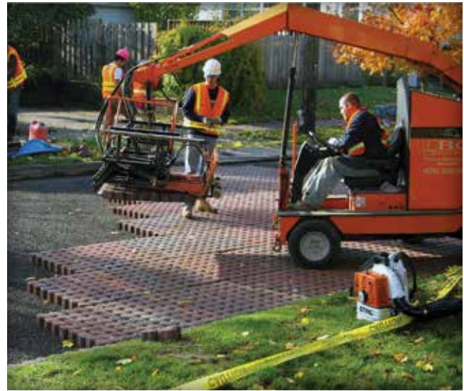
Figure 27 and 28. Mechanical equipment accelerated installation of a parking lot in Illinois and a street in Oregon.
