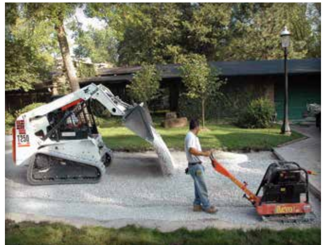
Figure 18. Compacting the berms along the perimeter and the PICP base
