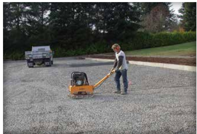
Figure 22. A 13,500 (60 kN) vibratory plate compactor is used on this ASTM No. 57 stone base.
