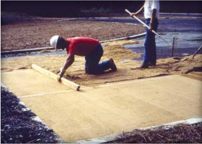
Figure 6a & 6b. Screeding the bedding sand.
