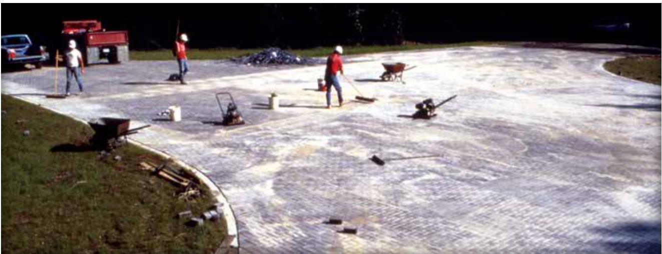
Figure 12. Excess sand swept from the finished surface will make the pavement ready for traffic.
